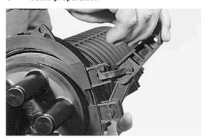
Open and remove the clamp. Remove the dome and the O-ring. Remark: take care with the O-ring and the sealing area ( surface ) on the base and dome ( avoid damaging ) . Clean only with clear water or with the cleaning tissue, if needed.
